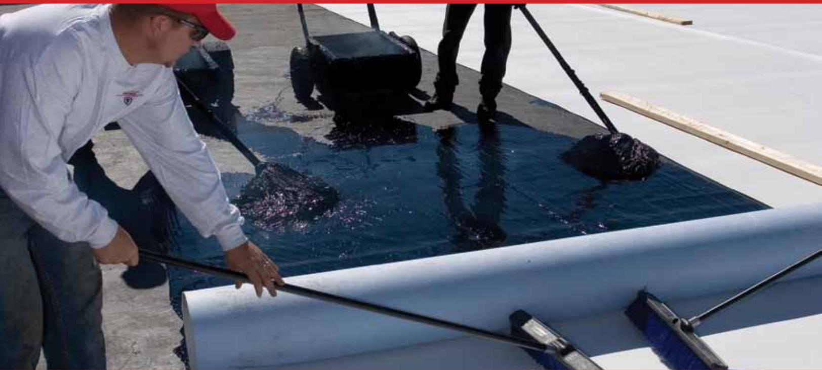
With a backing of eight-ounce, non-woven polyester fleece, Firestone UltraPly TPO XR offers an additional external reinforcement for remarkable puncture resistance. It combines the attributes of TPO with the great adhesion of fleeceback. The external polyester fleece enables installation with either hot asphalt or Firestone XR Bonding Adhesive. Plus, it provides excellent resistance to common rooftop chemicals and UV rays, through outstanding reflectivity, which can help you obtain LEED® points.
