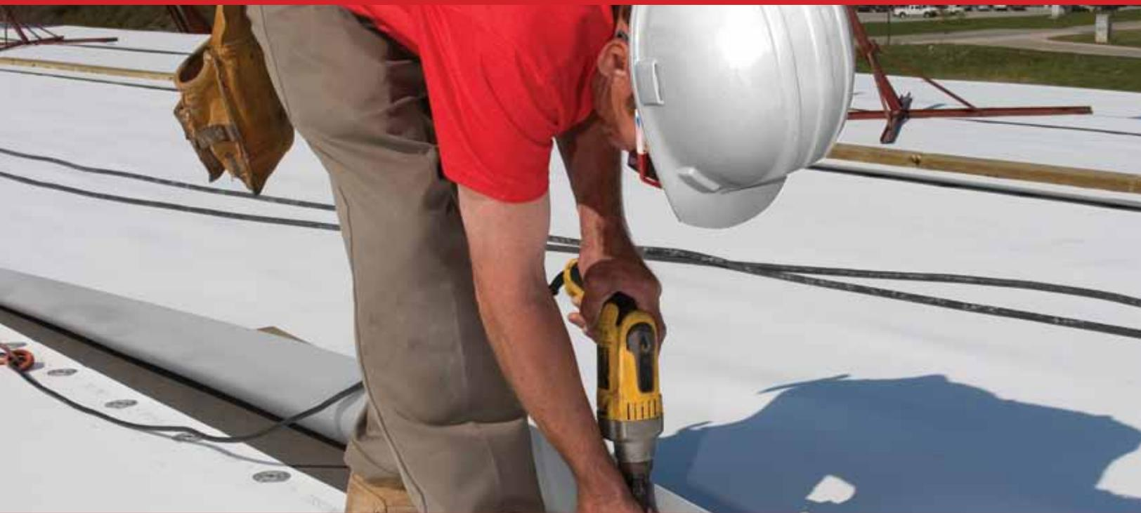
Light-colored roofs reflect UV radiation and improve a building's energy efficiency. ReflexEON TPO has the highest solar reflectivity of any TPO roofing membrane after 3 years of aging as tested by the Cool Roof Rating Council (CRRC). Its enhanced formulation provides uncompromised weatherability and durability year after year.
